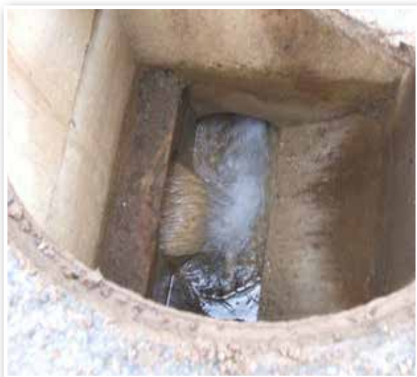
Surcharge hydraulique
